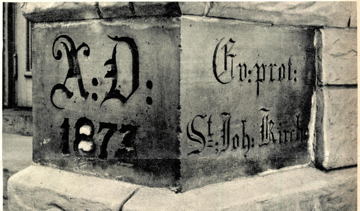
The cornerstone of St. John's Evangelical and Reformed Church, certifying how long this church building has been standing at Russell and Gratiot.
